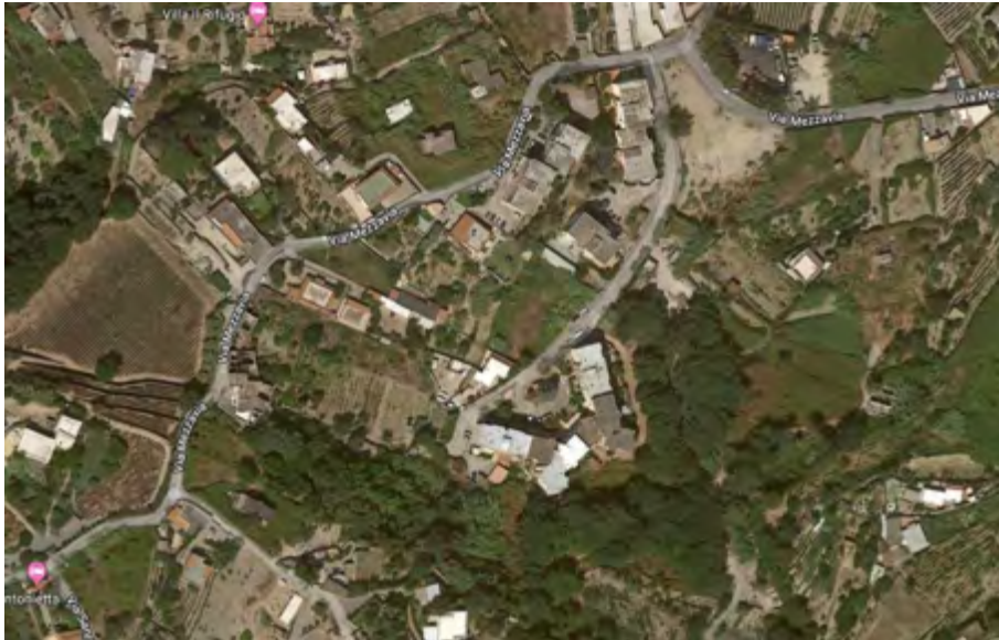
Fig. 2.2.4 – Ischia Island, Italy – Rural affected buildings in the 2017 earthquake – moderate damage degree
